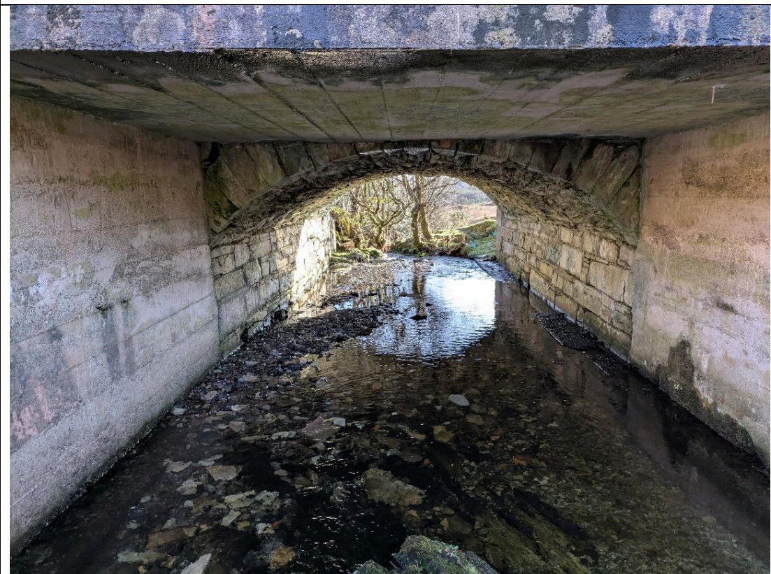
Plate 14-14: Original bridge (CH15) with adjoining modern concrete structure, facing east.
