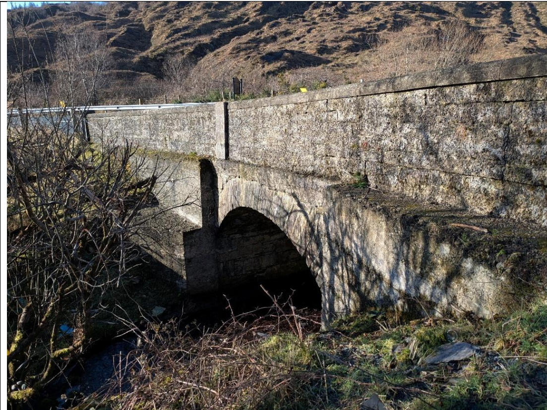
Plate 14-13: East façade of Carrigacorra Bridge (CH15), facing southwest.
