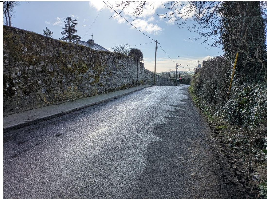
Plate 14-15: Upstanding boundary wall of Ballyhalwick House (CH20), facing south.
